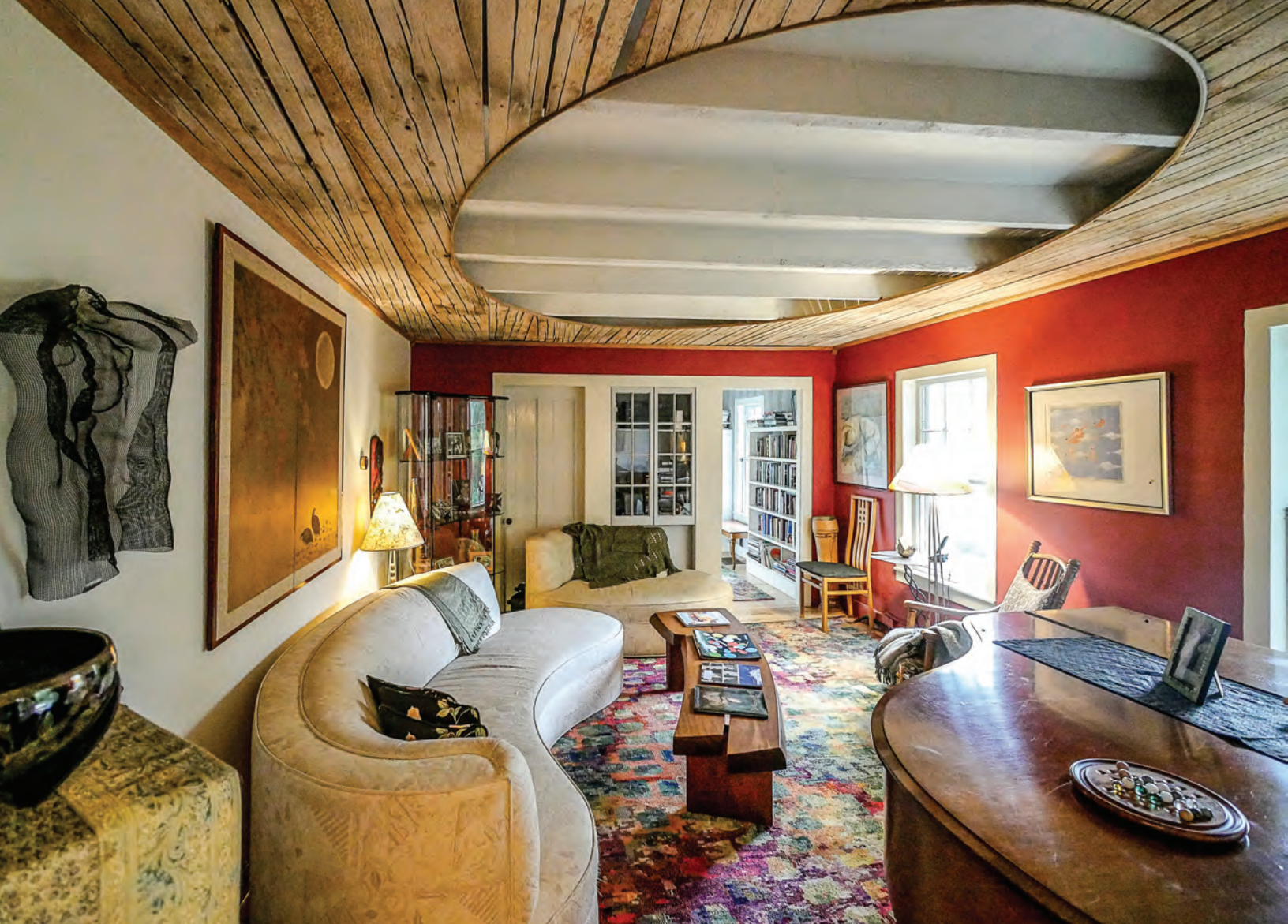
A puncture with a purpose: Once the drop ceiling was removed, it was decided the original plaster ceiling was far beyond repair, so it was removed and an elliptical cutout was carved in the split-lath ceiling to artfully expose the beams supporting the floor above.
