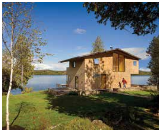
No sheetrock or other drywall construction is used in the camp because it is designed to weather severe changes in temperature, which cause expansion and contraction of materials throughout all four seasons, especially during the wintertime when the building does not see use.
