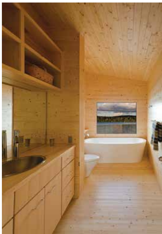
No sheetrock or other drywall construction is used in the camp because it is designed to weather severe changes in temperature, which cause expansion and contraction of materials throughout all four seasons, especially during the wintertime when the building does not see use.
