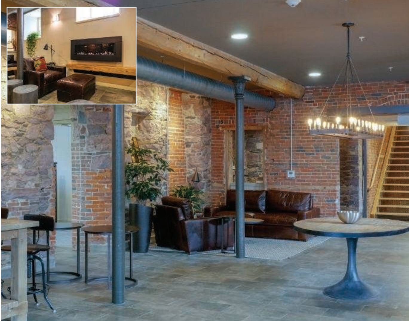
Stepping inside the new, handicap accessible main entrance, on the Lake Champlain side of Liberty House, site of the building's former basement. The rear of the building was regraded to allow for the new entry. The walls, a combination of brick and stone, were preserved as part of the spacious lobby/meeting area. Brick cleaning by Champlain Blasting Solutions. To the left is a separate bike/delivery entrance, bike cleaning area and a bike storage room. Inset shows the lobby's gas fireplace (from The Chimney Sweep). Staircase at rear from Hayley Custom Stair Co.
