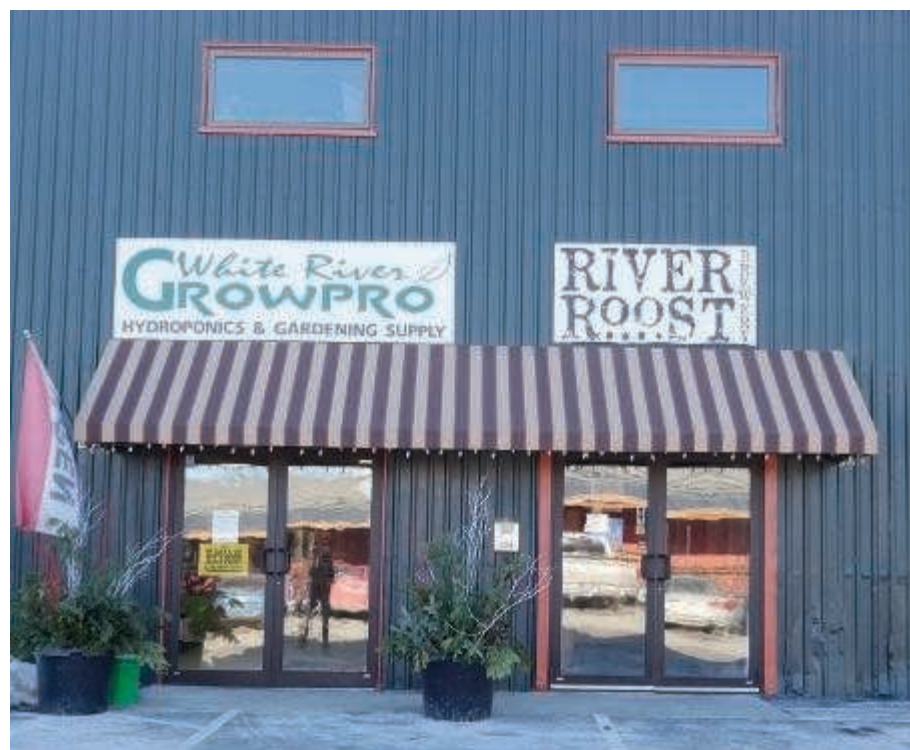
This newly constructed building, next door to Big Fatty's, was designed by Watershed Studio Architecture. In addition to a hydroponics store and brewery, it also is home to several offices.
