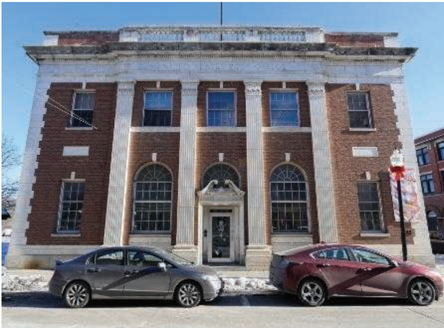
Above are two more historic buildings in downtown White River Junction that have been converted to modern use. The Gateway Building (top), the original home of Gateway Motors, now houses the Loewen Window Center of Vermont and New Hampshire, Watershed Studio Architecture and other businesses. The former post office building (bottom) is now headquarters to the Center for Cartoon Studies and Studio Nexus, among others.
