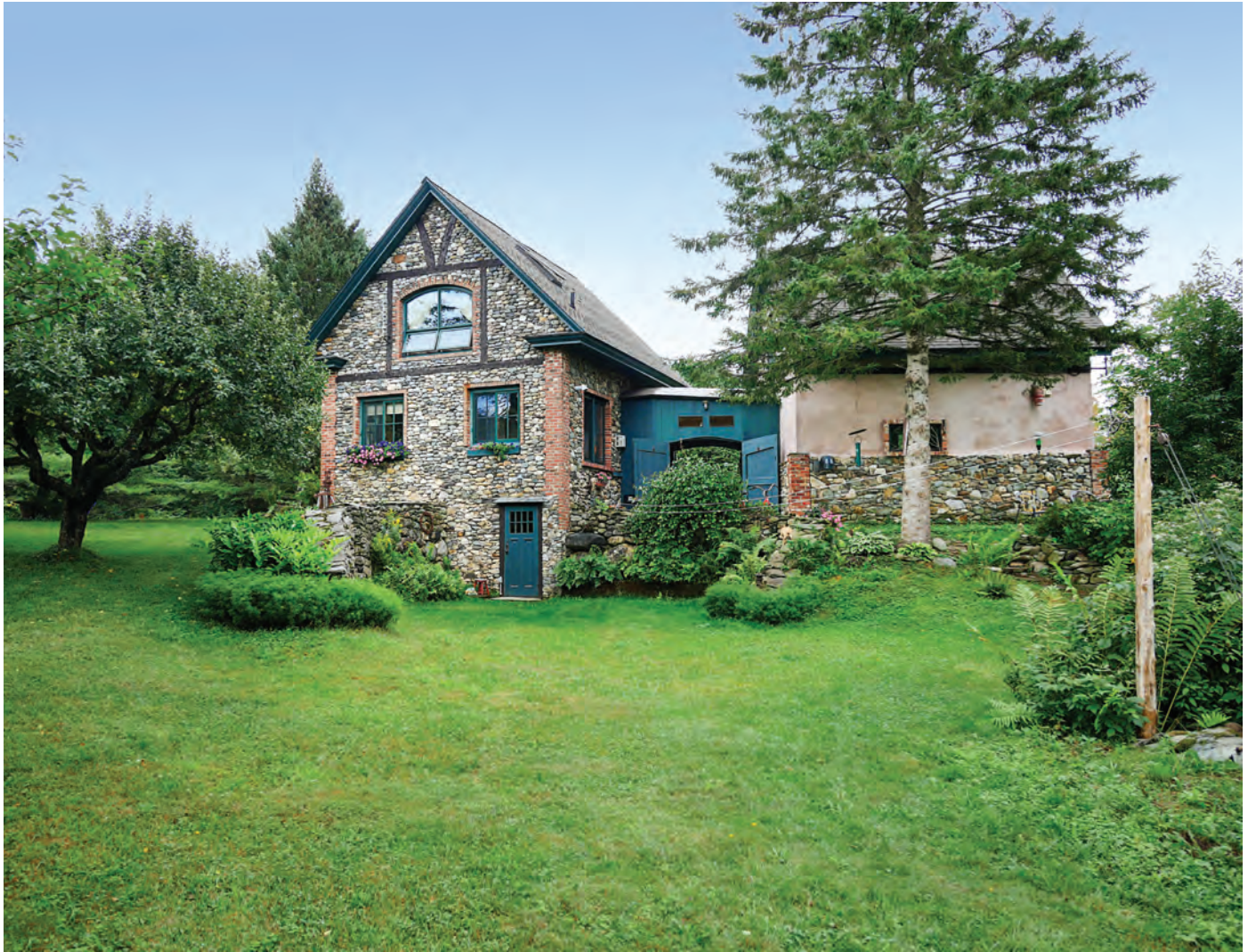
Lying between the two cottages, the covered and enclosed walkway sports two transom windows and opens to either side, plus the entrances of the two buildings.
